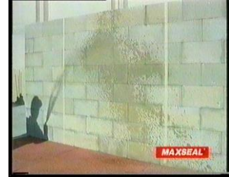
Wet surface before application.
