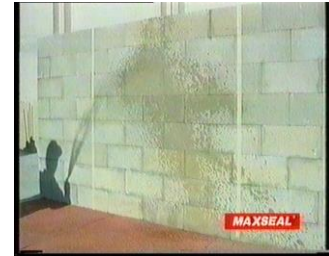
Wet surface before application.
