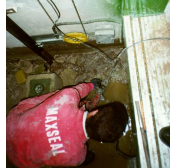
Cut out area and stop water flow using MAXPLUG
