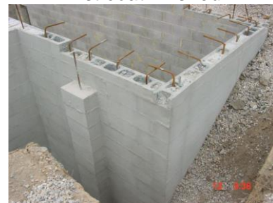
Second coat finished and partially backfilled.
