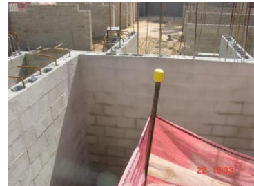
First coat finished.
