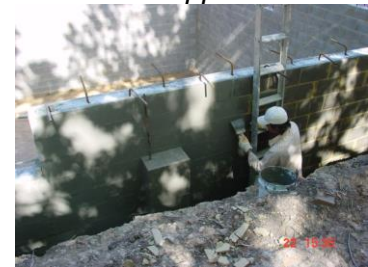
First coat of Maxseal Foundation.
