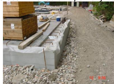
Backfill completed.
