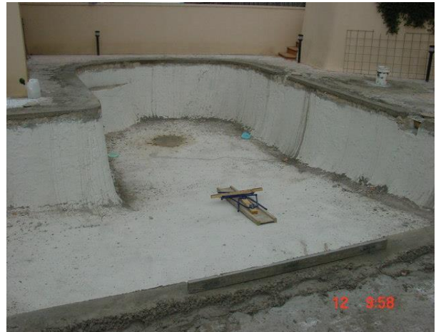
The bare concrete shell.
