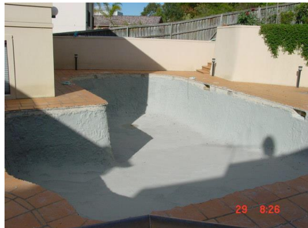
The pool after two coats of Maxseal Flex.
