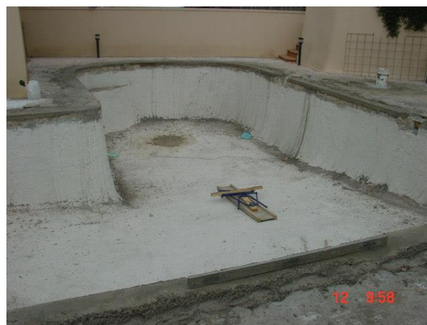
The bare concrete shell.
