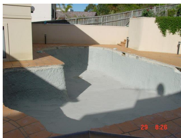
The pool after two coats of Maxseal Flex.
