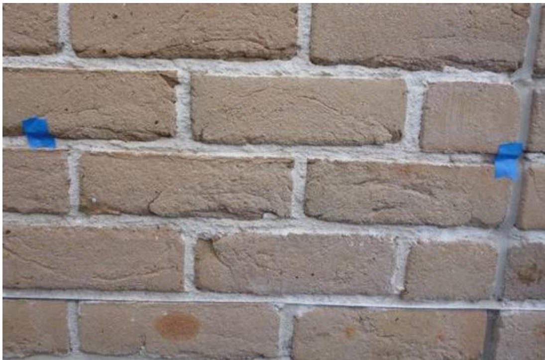
Figure 2. Joint chosen for sodium silicate trial (marked either end in blue)
