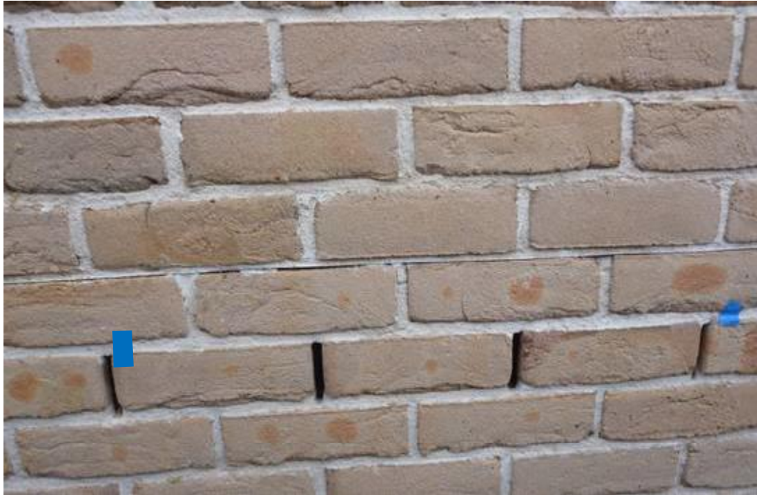
Figure 3. Joint chosen for Sealtight trial (marked either end in blue)
